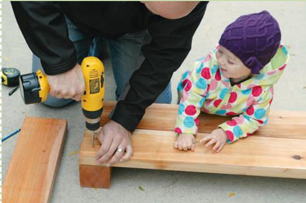
Attach two 3-ft.-long, 2-by-6 boards to the 4-by-4 corner posts.
